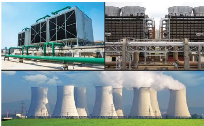
Cooling Tower Water Treatment Chemicals
